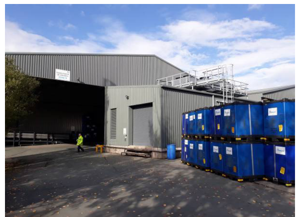
Current externally stored Plastic Preforms.
